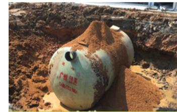
Installation of oil separator
